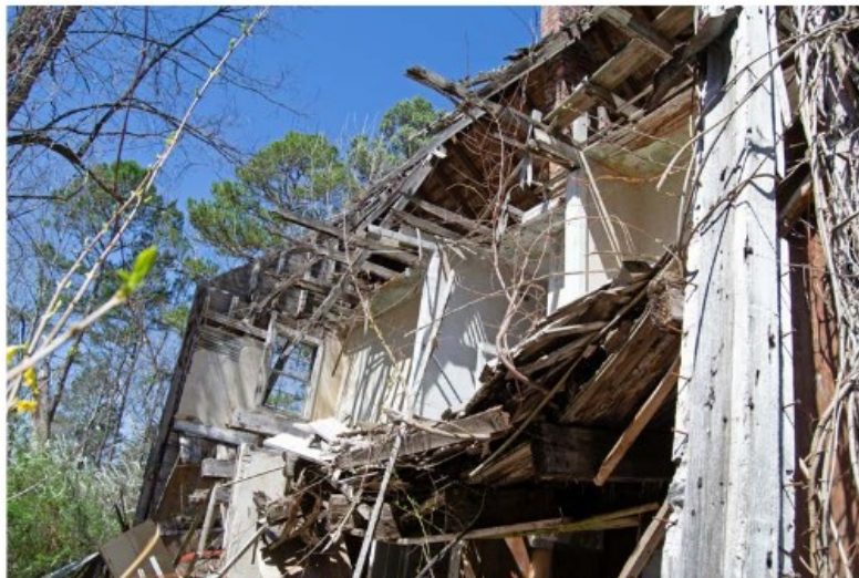
Photo 4: View of collapsed south wall, April 10, 2025.
